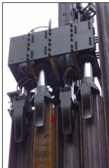
4 Cylinder Push-Pull on Liebherr LRB 255 piling rig installing U-piles - UK
