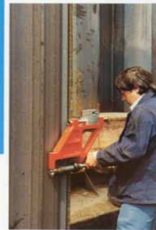
(left) Attaching the Pile Threader during a piling operation at Namur on the River Meuse in Southern Belgium. (right) Construction of a new quay at Inverness, Scotland. 1600 tonnes of Larsen B sheet piling were driven with the aid of the Pile Threader.
