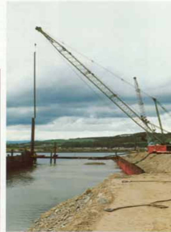
(left) Attaching the Pile Threader during a piling operation at Namur on the River Meuse in Southern Belgium. (right) Construction of a new quay at Inverness, Scotland. 1600 tonnes of Larsen B sheet piling were driven with the aid of the Pile Threader.
