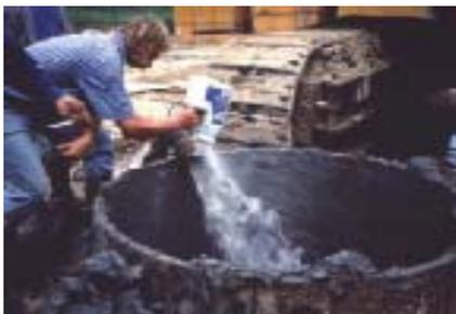
**Above:** SlurryPro CDP being added directly to a bored pile in Bangkok.
