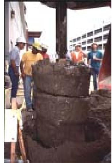
possible to slurry-drill with augers, even in sand and gravel, often eliminating the need to use a bucket. This feature can reduce drilling time, increase productivity and reduce slurry wastage.
